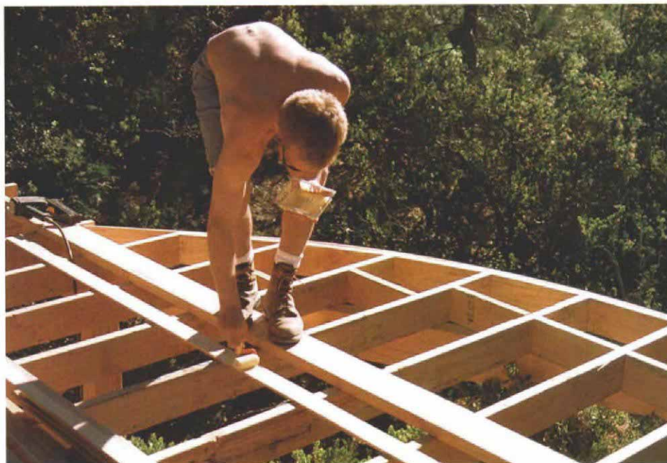
Waterproof glue and staples make quick, reliable laminations. The glue is applied with a disposable paint roller to ensure uniform coverage (photo above). A helper positioning the strips eases stapling them in the correct location (photo right).
