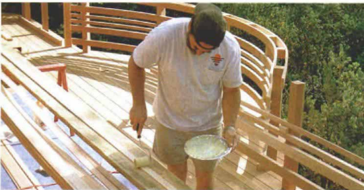
To support a narrow strip during glue up, an extra joist serves as a bench. This strip will be applied to the curved rail, partially completed in the background, then secured with staples while the glue sets.
