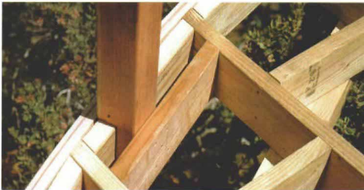
Blocking braces the newels. Because the newels are the forms for the railing, they must be braced to stay plumb while the railing is being bent. Bolts will reinforce this connection.
