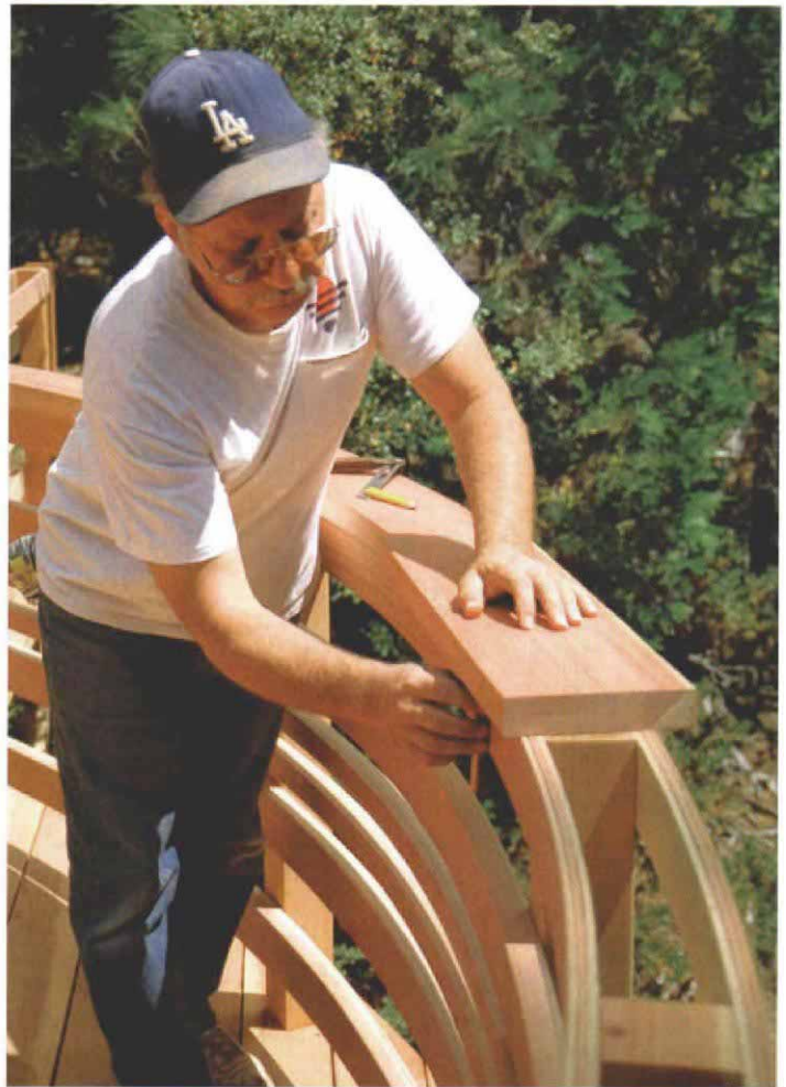
Pencil scribes the curve on the segmented 2x8 cap rail. Intermediate 4x4 blocks (foreground) support joints in the cap rail that don't fall on newels as well as provide blocking for the top bent rails.
