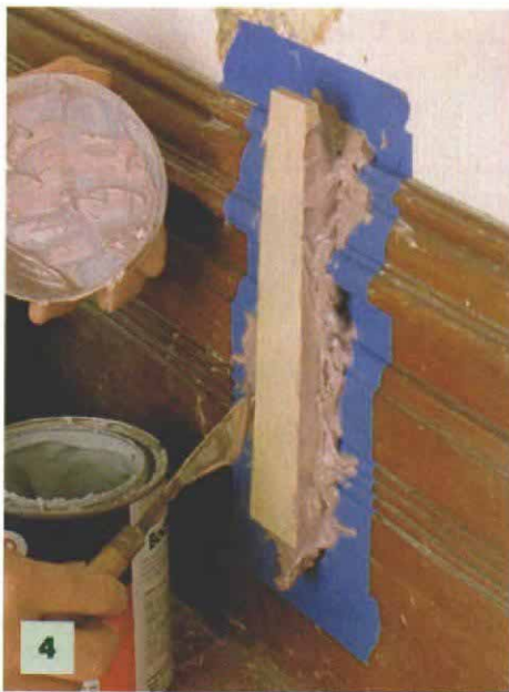
4. Reinforcing batten strengthens cast. A strip of wood pressed into the uncured body filler prevents the cast from breaking when it is removed from the baseboard.
