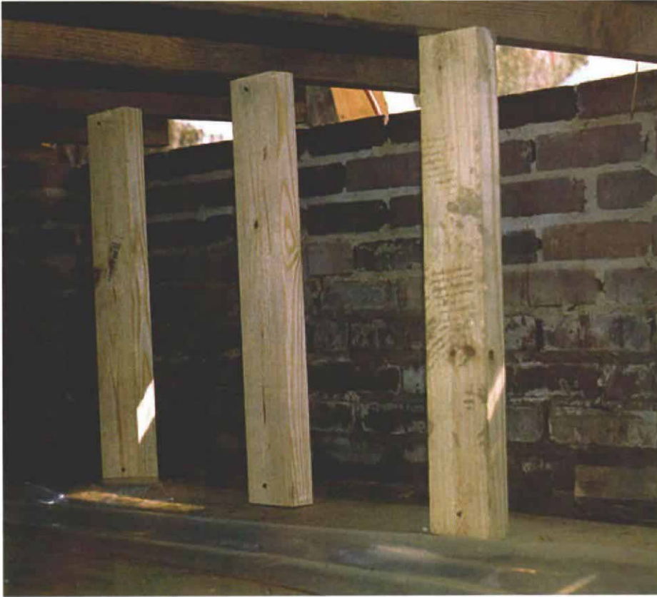
These 2x4 braces support the floor joists.
