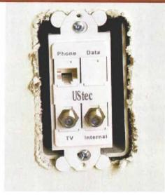
**Interface with this.** Really. This tech port is set up to handle phone and video. Other options are myriad, and a Decora-style plate finishes off the installation.
