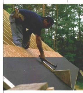
Scraps of 2x4 and oriented strand board are recycled into scaffold brackets, the first row of which is nailed on just above the bottom edge of the roof. A 2x10 plank nailed to the brackets creates a safe scaffold for sheathing and roofing. Successive rows of scaffold are installed at 54-in. intervals all the way to the ridge. These rows remain in place until the roofing above has been completed.
