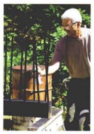
Painted spindles slide up and then down. Large nails partially driven into an old beam hold the conduit spindles as they receive numerous coats of primer and paint to protect them from the elements (photo above). As the final step, the author pushes the spindles up into the holes in the top rail and then down.
