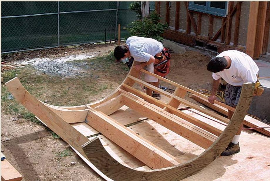
**Lack of plate overlap means metal straps must tie curved wall to straight. And yes, it would be safer to perform this operation on a ladder.**
