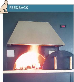
Wood-fired brick oven vents out and up. One of the kitchen's specialized appliances, the oven traps radiant heat in its dome and vents smoke and hot air through the door to a hood. The fire's ashes are pushed to the back of the oven and replaced with a pizza, a roast or loaves of bread. Photo taken at C on floor plan.
