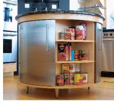
**Curved doors slide around the island.** A collaboration between the shop foreman and hardware manufacturer led to the design of the curved track that keeps the doors rolling smoothly. Photos taken at D and E on floor plan.
