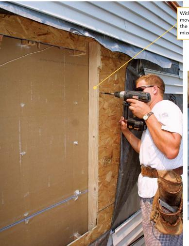
With the old studs removed, screws attach the new framing to minimize wall damage inside.
