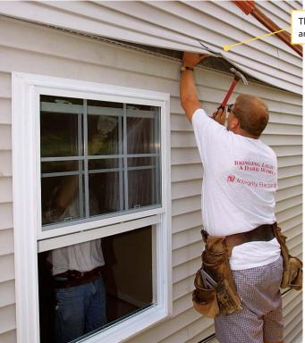
The siding is reinstalled and zipped back in place.
