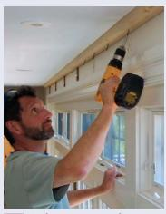
A cleat supports the valance. Screwed into the ceiling, the 2x3 creates enough space off the wall to house the shade and offers blocking for the face of the valance.
