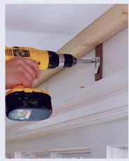
**Blocking guides the shade.** Mounting the hardware on ¼-in. blocking pushes the shade away from the wall to prevent it from hanging up on the casing.
