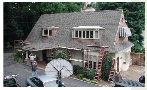
With the posts braced and in place, we installed the headers. At the end of the day, we covered the holes in the roof made by the new posts with aluminum flashing and plastic sheeting (top drawing, facing page).
