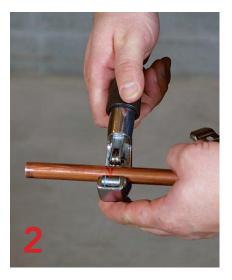
Cut it tight and square. To fashion the strongest bond, size the pipe to extend all the way to the back (the shoulder) of the fitting (top photo). Use a tubing cutter, rather than a hacksaw, to make a perfectly square cut (photo left); then ream the end of the pipe to remove the burr left by the pipe cutter (photo below).
