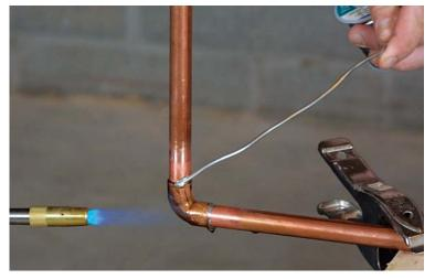
Color and flux tell you it's time. Continue to apply heat until the flux begins to melt and the copper takes on a shiny, iridescent appearance. Then touch the tip of the solder to the joint; if it's hot enough, the solder will pour in and encircle the fitting before it begins to overflow. When working with ¾-in. or smaller pipes, there's no need to drag the solder all the way around the joint to fill it adequately.
