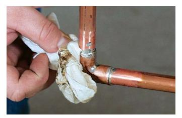
**10** Not just for show. Even if the pipe is to be buried beneath drywall, always wipe the solder with a rag before it has had time to cool. A bright, uniform solder joint between the fitting and the pipe is proof of a job well done.
