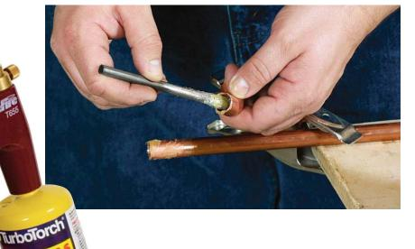
Apply flux to D deep-clean the metal. Brush a liberal coating of flux onto both surfaces (the flux removes minute traces of tarnish and etches the copper to promote adhesion with solder). To prevent contaminating the flux, close the cover tightly when not in use, and store the brush in a plastic bag.
