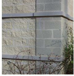
Smooth block meets rough block. Sandblasted-block piers at the corners frame fields of split-faced block. Narrow ribbons of concrete coping form subtle bands that delineate railing heights, thresholds, and sills.
