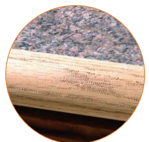
A half-round nosing softens the countertop edge.
