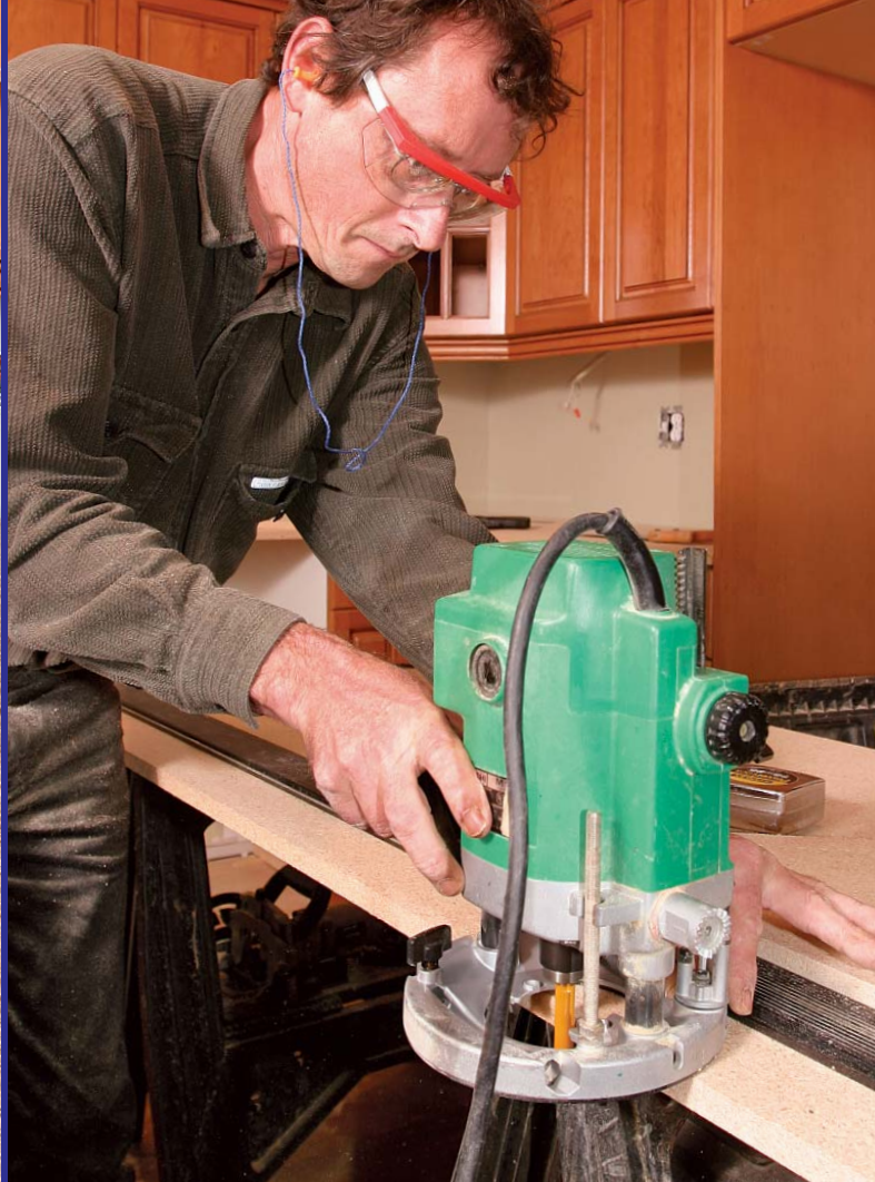
The substrate is critical. To ensure accuracy, the author fabricates the substrate where it will be installed. Here, he's truing a particleboard edge by guiding a router against a straightedge.
