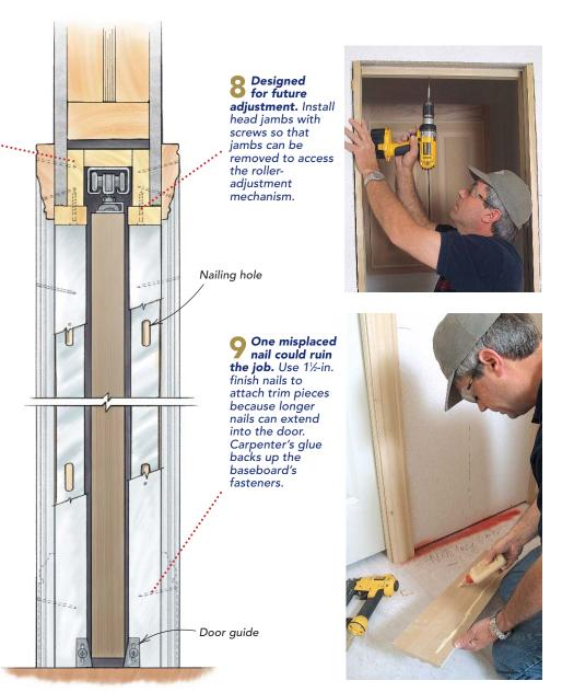
process. If the track is out of level, it may be impossible to get the door plumb or to keep the door in the opened or closed position.
