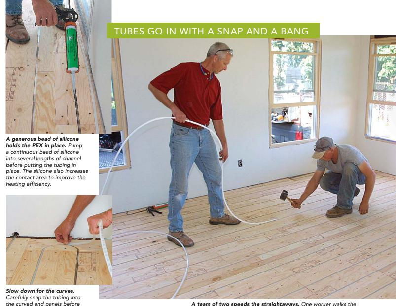
A team of two speeds the straightaways. One worker walks the PEX into place, and an assistant hammers it into the channel with a rubber mallet. Before the silicone dries, double-check to make sure all the tubing is seated properly.
