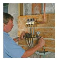
**Test the system with air.** Leave the pipes pressurized at 40 psi to 60 psi while installing the finished floor to warn of tube punctures from errant nails or construction debris.
