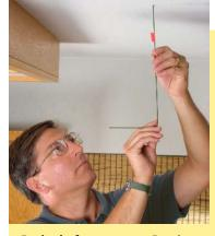
Probe before you cut. Bend a coat hanger to the radius of the fixture. Mark the depth of the fixture with tape. Spin the hanger as you push it into the ceiling to check for framing, ductwork, or pipes.
