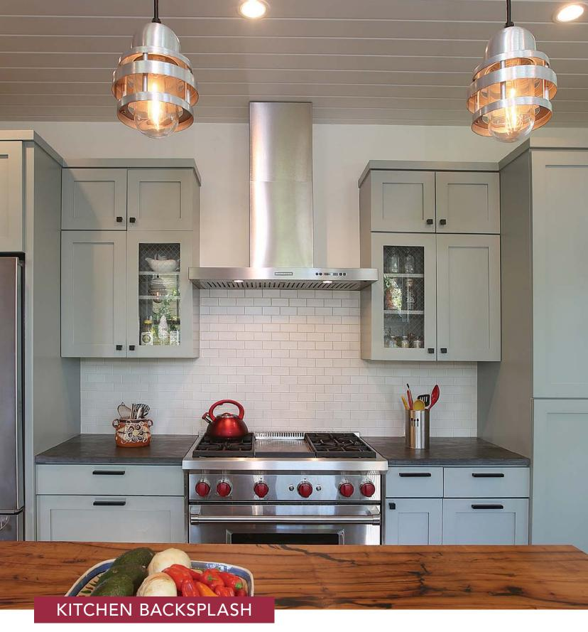
Compared to a shower or tub surround, a backsplash sees less water, which means that the substrate can be standard drywall, and mastic is an acceptable adhesive. Be mindful of the often long horizontal shape of the space, the number of cutouts needed for outlets and fixtures, and the possibility
