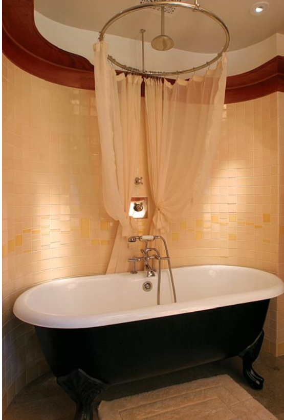
Curved tub, curved wall. Instead of square corners behind the tub, curved ones minimized incursions into the closet space on the other side of the wall. Photo taken at C on floor plan.
