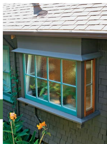
Shallow bay tucks under the roof. Protected by the roof overhang, the box-bay window extends just far enough from the house not to intrude into the adjacent pathway. Photo taken at B on floor plan.
