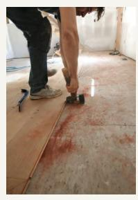
**Reverse direction.** Purchased separately, spline stock is like a long piece of double tongue that can be cut to length and seated in a board to bring two groove sides together.
