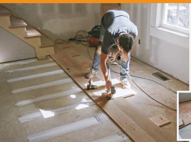
And they're off. Production begins with skip troweling glue every 2 ft. or closer. From this point forward, board selection is driven in part by where butts might appear, so as to create the most cohesive appearance possible. To keep things moving, butter ends from a neighboring line of glue, making these joints just as strong as end-matching. Backcutting with a 2° bevel ensures a snug fit.
