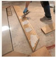
bottoms. Like the floorboards that will be installed across the rest of the room, the picture-frame boards are secured in part with Bostik's urethane-based hardwood-flooring adhesive.
