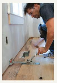
**Flooring jack.** The flooring stapler won't fit close to the wall, so the second-to-last row of boards is held tightly in place with a flooring jack and then face-nailed sparingly.
