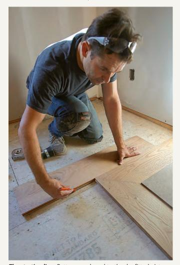
The starting line. Butt a scrap board to the dry-fitted picture frame to establish a line of reference. Measure the distance from the line to the wall it runs parallel to, and check the wall for square. Repeat the measurement at the other end of the room, and snap a chalkline between the marks.
