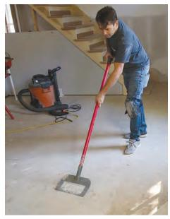
A clean slate. Thorough inspection of the subfloor helps avoid oversights or surprises once installation begins. Be sure to address any voids or squeaks, and shim, scrape, or grind for flatness. Here, a roofing scraper removes drywall mud.
