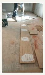
**Starter course.** Butter the first board with glue, and then secure it in place with a flooring nailer loaded with 2-in.long 15-ga. flooring staples. For <sup>3</sup>/4-in.-thick plank floors, the nailing schedule is every 4 in. to 6 in. and 2 in. from the ends.
