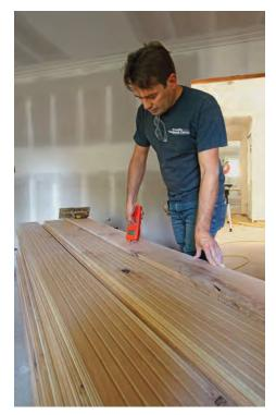
Measure moisture. Ideally, the flooring has been on the job site to acclimate for at least three days. Before installing, use a moisture meter to make sure the flooring is within ±2% of the subfloor. This will avoid problems such as gaps and buckling down the road.
