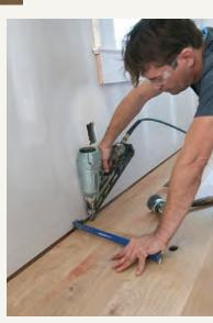
**Expansion gap.** Leaving a <sup>3</sup>/<sub>4</sub>-in. gap between the flooring and any obstructions allows the planks to expand with moisture fluctuations.
