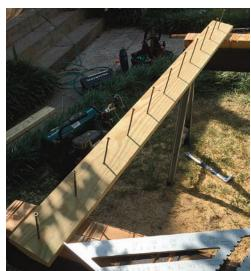
Pilot holes are a must. KDAT lumber is dry and prone to splitting, so it's crucial to lay out and drill pieces before assembly. Exterior wood screws are driven from the flat side of the subrail, where they will later be concealed and protected from the weather by the top and bottom rails.
