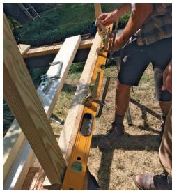
A level for alignment. The birdsmouth joint between baluster and subrail helps with alignment, but doesn't guarantee it. Start each rail section by fastening the two outermost balusters, and then clamp a level against their faces to create a guide for the placement of each additional baluster.
