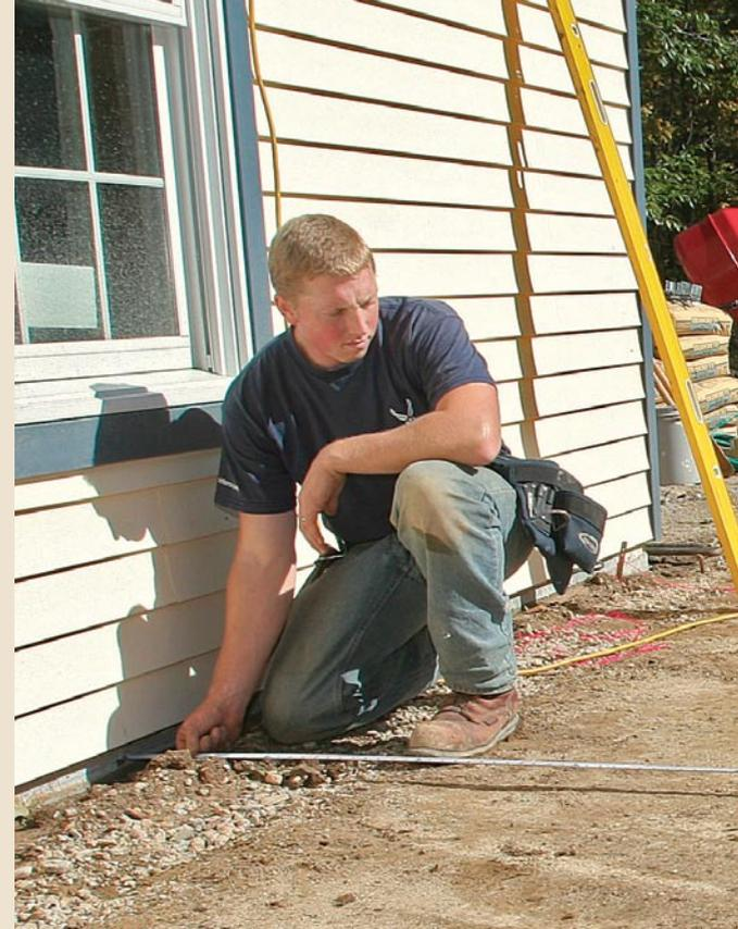
I found that dividing the rim joist into three sections gave me a span of roughly 5 ft. 4 in., which came out to four piers. Even though my double rim joist could span 8 ft., I chose to use a 5-ft. 4-in. pier spacing to minimize the pier diameter.
