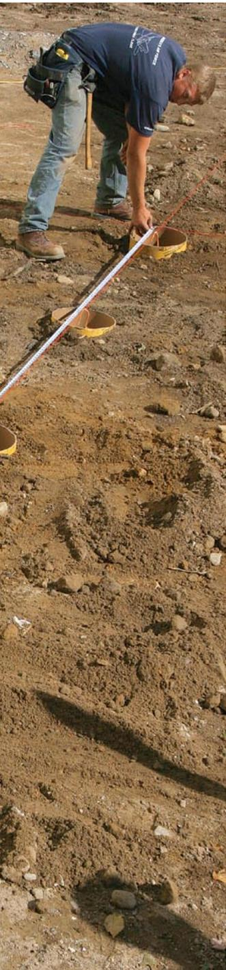
**3 A shovel makes up for bad aim.** Fill the tubes with concrete until it reaches the nail. The concrete should be just slightly on the wet side, about the consistency of thick oatmeal. As the concrete is poured into the tube, a helper uses a shovel to agitate the mix every 8 in. to 10 in. to work out air pockets.
