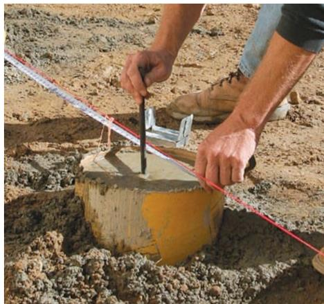
**4 Place anchor bolts accurately.** Once all the piers are poured, I go back and insert anchor bolts in the center of the piers. I measure from the line running perpendicular to the house to set anchor bolts accurately. Be sure to leave the threads high enough so that a post base, washer, and nut can be added later.
