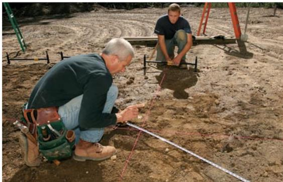
**3**  **$A^2 + B^2 = C^2$ .** Pulled diagonally from the foundation, my tape forms the hypotenuse of a right triangle. A helper shifts the line that extends from the house to intersect with the right measurement, identifying the center of the far-corner pier.
