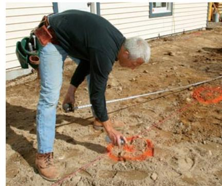
**4** **Mark piers with paint.** Measure the remaining piers from the far-corner pier. A dot marks the centerpoint, and a rough circle highlights where to dig. Pull the stringlines and prepare to dig, but keep the batterboards in place.
