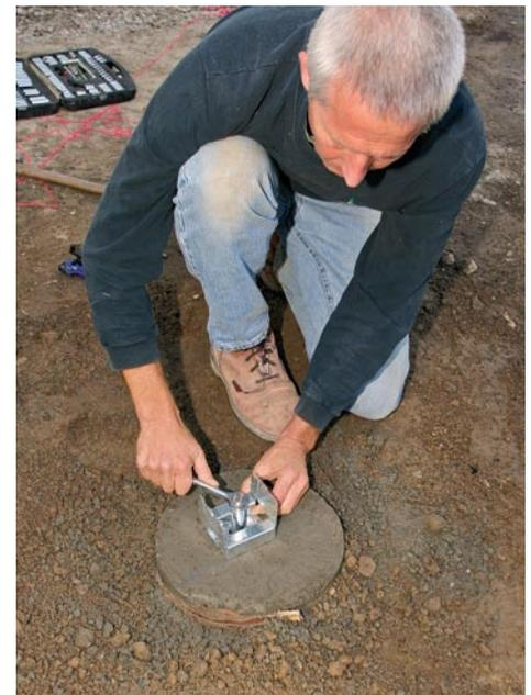
**5 Adjustable post bases allow for final tweaks.** After the concrete is cured completely, I attach adjustable post bases. I like to use Simpson ABA-style bases because they allow me to fine-tune the post location after the post is attached.
