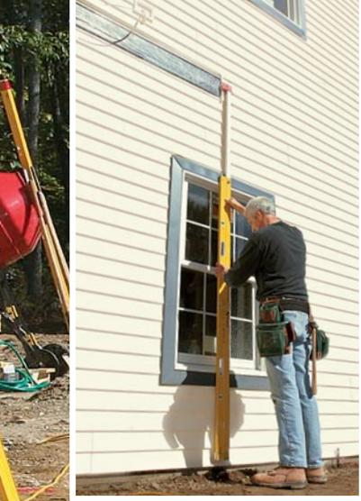
**1** **Plumb down from a high ledge.** With a Stabila plate level ([www.stabila.com](http://www.stabila.com)), I carry one end of the ledger down to the grade. I drive a stake into the ground here to anchor a line that will run perpendicular to the house.
