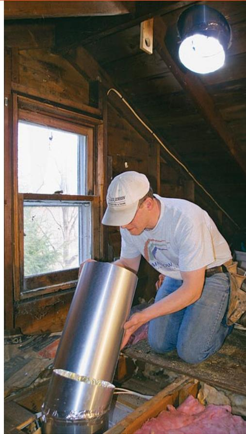
**Connect the tubes.** The tube extensions fit together and are sealed with tape supplied with the kit. Once the tape goes on, the tube is fairly rigid, but most manufacturers supply machine screws to hold the tubing together.
