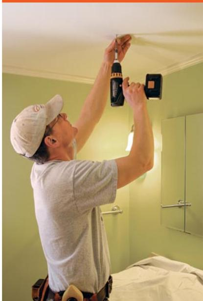
**Locate the center of the light, and drive a screw through the ceiling. Get some reference points by measuring from an outside wall or ceiling light so that you can find the screw easily when you are in the attic.**
