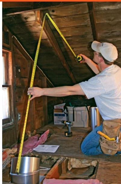
**Clear away the insulation and deal with any obstructions like wiring or ductwork. Use a tape to check angle and length. Before putting a hole in the roof, make sure you have enough tubing. Send a screw through the roof, and again, remember to get some reference points before you go on the roof.**
