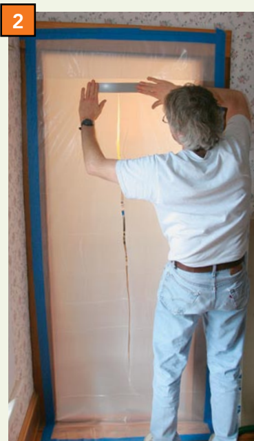
2 Apply strips of duct tape to reinforce the slit in the plastic and to keep it from widening as you walk in and out through the airlock.
