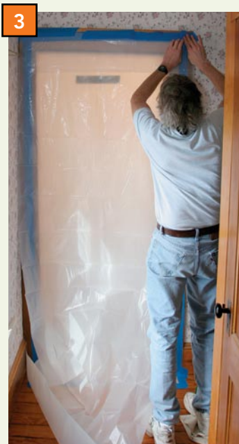
3 A second sheet of plastic covers the first, but it is taped (or anchored with a furring strip and screws) only to the head casing so that it can hang loosely.
