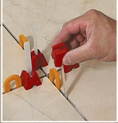
Cap the strap. Place the special cap that allows the strap to be pulled up, but captures it so it can't move backward.
