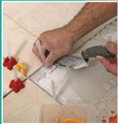
Slip in the strap. Lift the tile slightly with a margin trowel to help keep from pushing mortar out with the strap.
