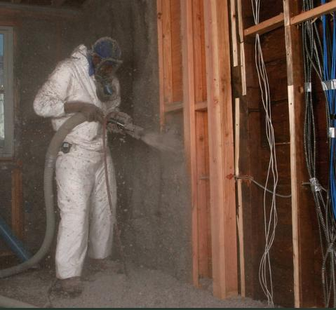
must first air-seal any penetrations (can lights; holes around pipes, ducts, and cables; and the gap around chimneys) before blowing. Loose-fill settles about 10% after installation, so this must be accounted for when planning how deep to blow in the insulation.
