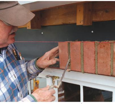
**Drain the brick.** Water needs a way out. Soak  $\frac{1}{4}$ -in. dowels in water overnight, and set one in a mortar joint every foot or so. In an hour or two, rotate and pull out the dowels.
