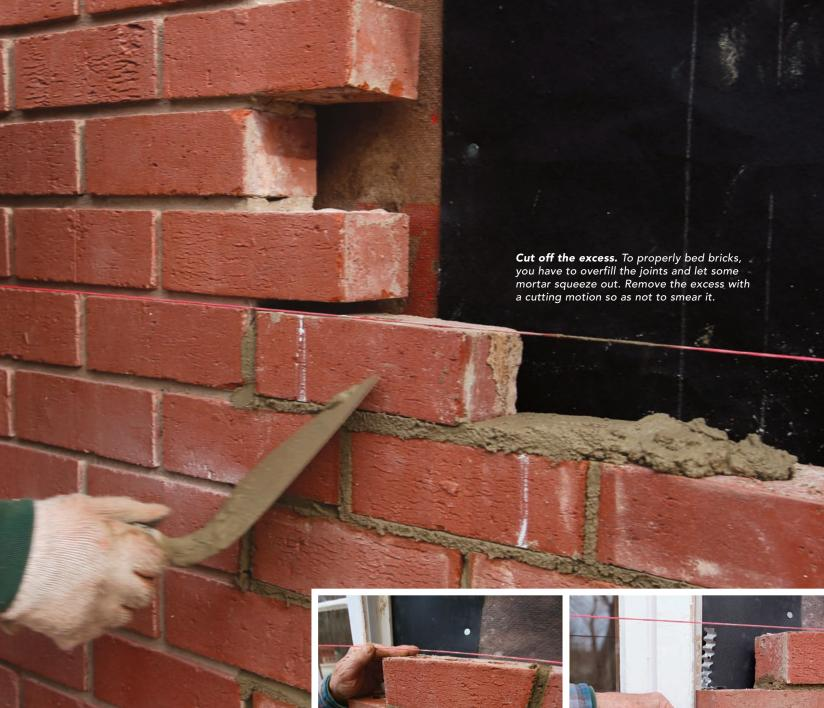
faster in hot, dry weather than on cool, damp days. The existing joints on this house were simply recessed about 5/16-in. deep. To match that joint profile, I used a wheeled joint raker (photo near right), setting the nail (a regular 10d common nail) to rake out the mortar to the same depth as the joints on the existing brick wall. After raking the joints, I used an old paintbrush to sweep away the crumbs.
