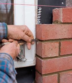
Work in from the corner. A joint raker won't fit where the brick returns to the window, so a tuck point is used instead. To make a crisp, mortar-packed angle, work the mortar away from the corner.
