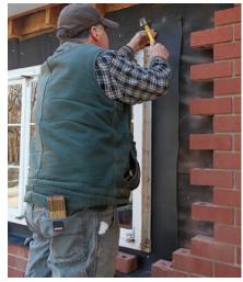
Foam for a gap. To hold the bricks a consistent 1/8 in. away from the window and provide a backer for sealant, apply foam weatherstripping along the window sides and beneath the sill, about <sup>1</sup>/<sub>4</sub> in. back from the face.
