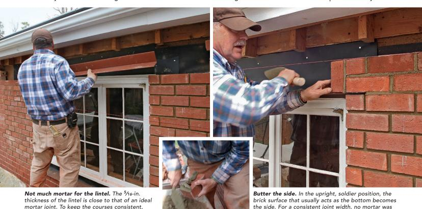
**Brick-spacing rules** The total height of brickwork is adjusted via the thickness of the joints. Thicker joints make brickwork taller (or wider, in the case of bricks laid sideways like in sills or soldier courses), while thinner ones make brickwork shorter (or narrower). A brick-spacing rule
