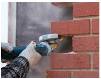
Grind away. A grinder removes mortar without shocking surrounding bricks, but this tool can only reach the outside edges because it doesn't fit between bricks.
