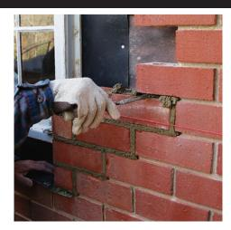
**Pack in mortar.** Fill bed joints between the new brick and the half of the brick above using a <sup>1</sup>/<sub>4</sub>-in. or <sup>3</sup>/<sub>8</sub>-in. tuck pointer. Put a mound of mortar on the brick, and push it in until the joint is packed solid.
