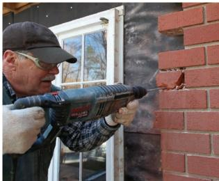
Break the brick. To take pressure off the surrounding brick, first weaken the mortar by drilling a series of holes all the way through the joints, then break the brick by drilling holes from the outside in.
