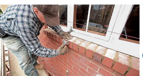
The final raking. To prevent blowing out the corners, rake the joints from the bottom halfway up, and then finish by raking down from above.
