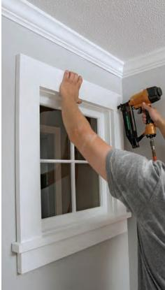
In and trimmed. With the opening prepped, set the window in place—centered and double-checked for plumb—and then fasten through the casing with finish nails. The unattached casing is then installed on the opposite side and fastened, covering the wall surgery completely.
