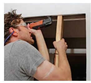
Retrofit a rough opening. Any studs that extend through the new opening must be accurately cut back. Measure 1½ in. from the cut edge of the drywall, mark a line across the face of the stud, then make the cut at an angle away from the line using an oscillating multitool. Toe-screw the new sill and header to blocking added to either side of the opening and then into the angled cut, which ensures that the new 2xs won't be thrown off by out-of-flat cutting.
