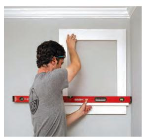
**Trim as a template.** After holding up and leveling the unattached trim assembly on the wall, trace around its inside perimeter. Then, add a little more than the thickness of the jamb to the scribed line to find where to cut back the drywall. Cut the opening with a new, sharp utility-knife blade, making several passes.
