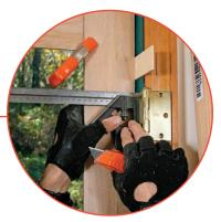
The template doubles as a story pole. Using a combination square and a utility knife, transfer each hinge location precisely to the template.
