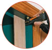
Modify the template for a bowed jamb. If the jamb is not straight, use a compass to scribe the jamb's irregularities onto the template. Shave the template to the scribed line with a block plane, and complete the assembly. The same technique can be used to fit doors to warped or worn thresholds.
