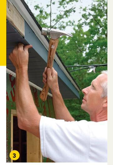
Install the aluminum fascia with color-matched nails. I bend  $\frac{1}{2}$  in. of the first piece around the end of the subfascia with a hammer (see the arrow on photo 6). Then I slip the aluminum fascia behind the drip edge. I nail the aluminum fascia about 2 ft. on center, alternating high and low, and pushing the lower edge against the soffit as I go. Overlap adjacent pieces by 1 in.
