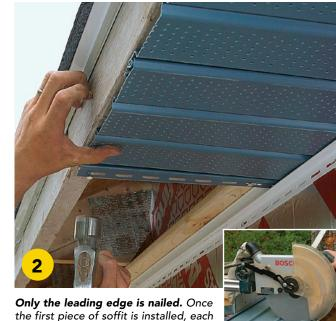
consecutive piece snaps into the previous one. I nail the leading edge to the underside of the subfascia and to the furring strip above the F-channel with 1½-in. roofing nails. Use a plywood blade installed backward to cut the soffit material.
