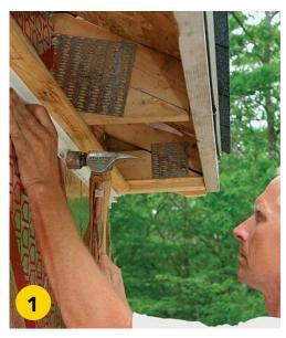
Install the F-channel flush with the bottom of the subfascia. I hang the subfascia ¾ in. down from the truss tails to widen the fascia, so I nail strips of furring to the bottoms of the tails. I nail the F-channel just below the furring with 1¼-in. aluminum roofing nails 16 in. on center. Leave the nails ¾2 in. proud (the thickness of a dime) to allow for thermal expansion.
