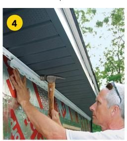
If you want a vinyl frieze board, use a starter strip. After the corner piece is up, I install the starter strip just below the F-channel using the same nailing technique I used when installing the F-channel.
