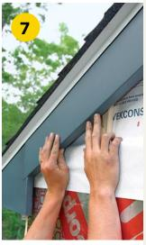
**Aluminum runs up the rake.** I bend a piece of aluminum to wrap around the soffit return and slip it behind the drip edge (photo left). An extra bend in the rake hooks the bottom of the subrake (sidebar right), so I nail the aluminum only at the top. Overlap the rake pieces by 1 in. to shed water.
