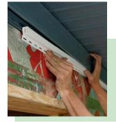
This house is ready for vinyl. Although the eave approach in this article can be used for just about any siding application, I installed vinyl siding on this house. A vinyl termination strip (shown far left) slips into a rabbet in the vinyl lineal and secures the ripped edge of the last course of vinyl siding. Rigid-foam insulation installed over sheathing increases the wall's R-value. (For more information, see FHB #181, p. 88.)
