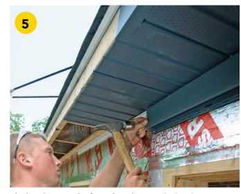
The lineal mimics the frieze board. I snap the lineal in place and nail it every 16 in., again leaving the nails proud. The lineal finishes the eave and provides a rabbetlike groove into which siding can terminate.
