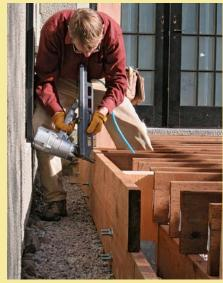
Toenail joists to beams. Straight joists mean straight lines of screws in the decking. After toenailing the joists on the layout, I add blocks around the posts to catch the ends of decking boards (inset).
