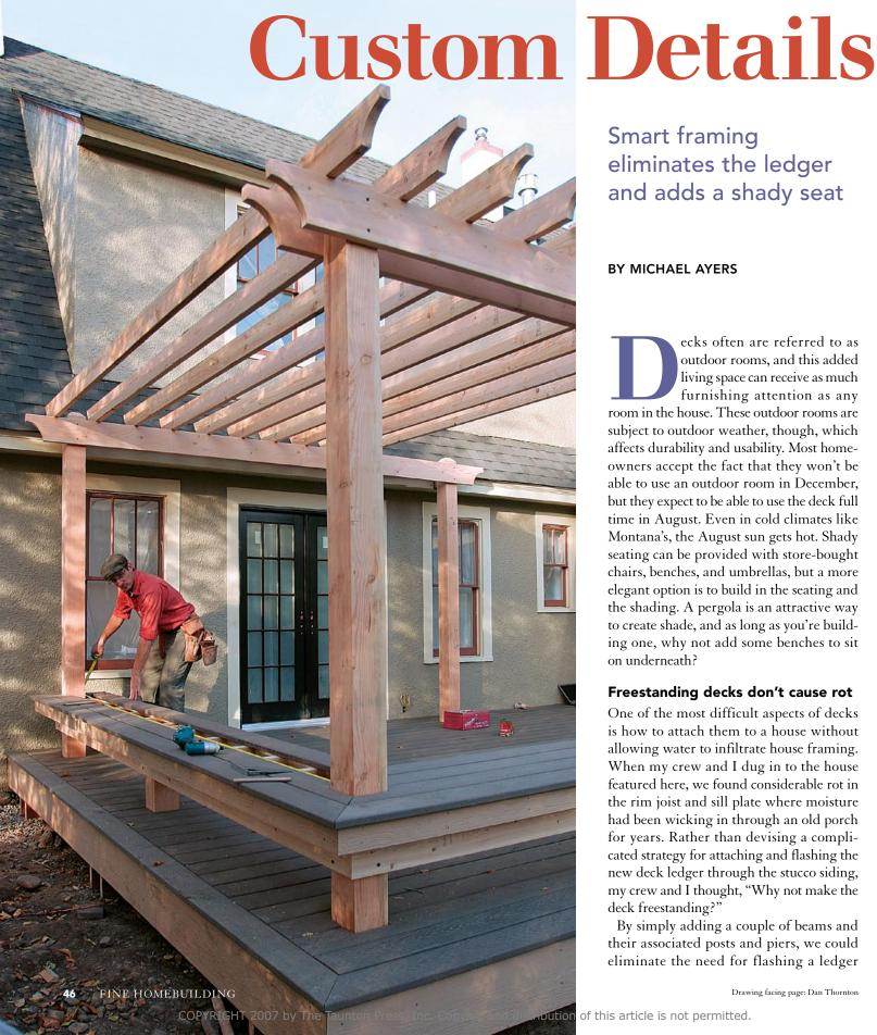
**Smart framing** eliminates the ledger and adds a shady seat
