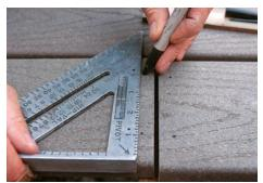
**Tip: Speedy screwing template.** If you don't want to place screws by eye, mark your Speed Square with a felt-tip pen; slide the square along or mark the boards individually.
