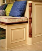
**Columns warm the color scheme.** Basing the design on a profile taken from architect Edwin Lunde, who remodeled this particular house 70 years ago, Jon's shop turned a clearfinished quarter column of mahogany to punctuate the transition between an end panel and an adjacent built-in seat.
