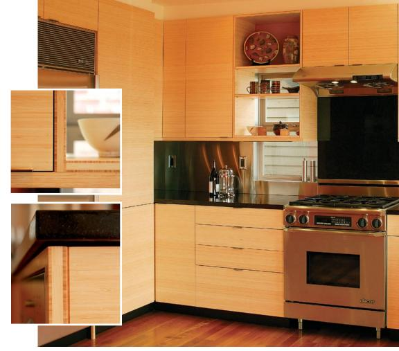
**The material speaks for itself.** Applied over stock cabinets, the bamboo plywood's laminations (top left) create a decorative edge that doesn't need edgebanding. The base cabinet's end panel (above left) is highlighted by a narrow kerf cut where the panel meets the unbanded edge of the front panel.
