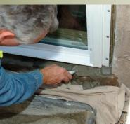
Slope the sill to help shed water. With the window in place, I mix a small amount of concrete and apply it under the lower nailing flange. Slope the concrete just enough to ensure that any water running down the window drains away from the opening.
