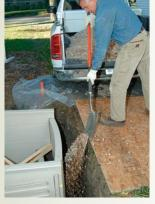
4. Two-tiered back panels double as steps. With the two sides anchored to the foundation wall, I attach the two-tiered back panels, which double as steps for climbing out of the hole in case of an emergency. After bracing the window well so that it stays square, I evenly backfill the hole with gravel to provide adequate support and drainage.
