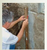
2. Measure and mark for the new opening. After transferring the dimensions of the window well to the foundation wall, I use a level to scribe a plumb line so that I can accurately position the pilot holes needed to attach the L-shaped metal flanges that hold the window well to the foundation wall.
