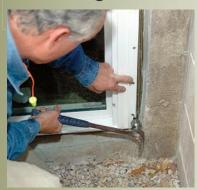
Corrosion-resistant nails are a must. This is a below-grade installation, so I fasten the window to the pressuretreated bucks with stainless-steel nails.
