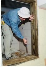
Fill the voids and frame the opening. With the sides of the opening smoothed out, I use bag-mix concrete to fill the cores in the exposed block at the bottom of the opening and to level any inconsistencies in the block. Then I frame the opening with pressure-treated bucks and seal the exterior joint between the new wood and the existing concrete with urethane caulk.
