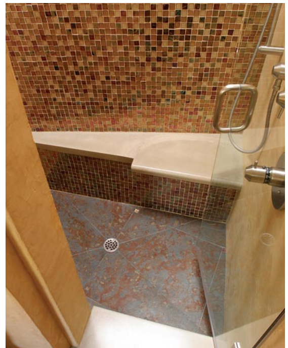
Just enough bench. A triangular cast-concrete shelf in the shower makes a convenient spot to sit and soak. Both bathroom and shower floors are slate, offset at the corners to include glass-tile insets. Photo taken at B on floor plan.
