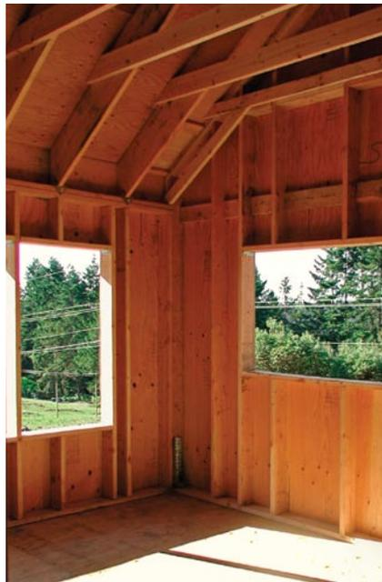
**Look! No headers.** Traditional framing (left) uses a lot of unnecessary wood. Optimum-value engineering (OVE; right) relies on careful structural analysis so that studs and headers are used only where they're needed. That means less wood, more insulation, and reduced thermal bridging.
