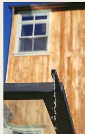
**NATURAL IRRIGATION** Runoff from the front-door overhang is conducted into two large planters, minimizing the need for watering. Rainwater from the roofs of the house and garage is stored in underground cisterns for irrigating the gardens.
