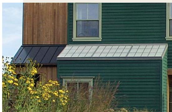
**DIFFUSED LIGHT FROM ABOVE** The roof of Larry's home office (and of several out-buildings) is made of Kalwall, a translucent, highly insulated building panel. The bright but diffused light that comes through the roof reduces the need for electric lighting.
