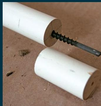
Longer balusters are required for certain parts of the stair. If you're lucky, your supplier has anticipated this and sent a few extralong balusters. If not, you can order one and wait a week to finish the handrail, or you can stretch one like this. Drill a pilot hole, and drive a 2-in. drywall screw into the end of a baluster. Grind off the head of the screw, glue and thread on a matching scrap of tapered end, then sand it flush.
