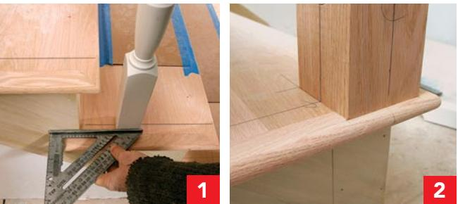
dle than a full-length piece, and as I work through marking and cutting the gooseneck assemblies, I might connect and disconnect an easement several times. I measure for and assemble the upper gooseneck first to establish the balcony newel-post height. Then I move on to measuring and cutting for the landing newel post. The process is the same for the balcony newel. I attach the gooseneck assembly to a straight rail and position it to measure the post height.
