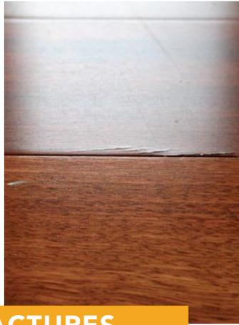
**Small cracks can be filled.** A board with cracks in its face doesn't always need to be replaced. The board shown here may be repaired with a touch-up kit.
