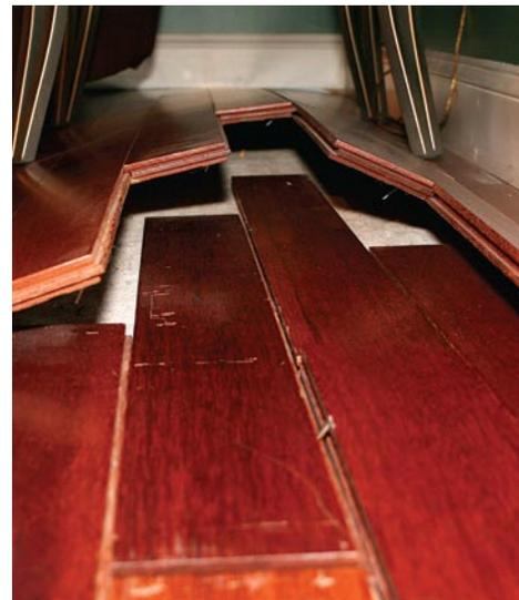
**Boards buckle if they can't expand.** When floorboards aren't acclimated or are exposed to lots of moisture, they can crush together and lift off the subfloor.
