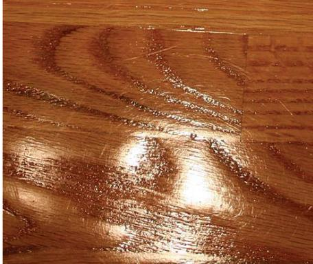
**Sloppy sanding shows.** Using a worn sanding screen to sand between coats of finish can leave spiderweb-like defects in floor finish.
