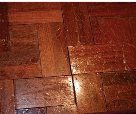
**Don't always blame the dog for fast-wearing floors.** *A worn floor lacks sheen and evenness in color. Poor finishing techniques can be the cause as much as family pets and household abuse.*
