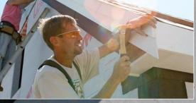
To hide any irregularities in the rake boards, such as gaps caused by rafter crown, I install a double member. I measure up from the bottom edge of the rake boards and snap a chalkline to guide the installation. If I know there will never be a gutter, I use a beveled double member on the fascias as well. If you use this detail, remember to allow visually for the coverage of the drip edge when sizing it.
