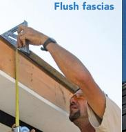
The fascia boards should never project higher than the plane of the roof. Depending on the roof pitch and the width of the trim board, you might be able to drop the trim a bit, tuck the top under the roof's drip edge, and still manage to get the right reveal on the soffit. In this case, I had to bevel the top edge of the fascia.
