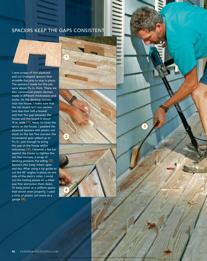
boards. (On this project, I used decking that was kilndried after treatment, or KDAT, so I needed to establish uniform gaps between the boards.)
