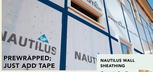
Georgia-Pacific's new sheathing, Nautilus, consists of its OSB product with a woven housewrap glued to one side. It's meant to be installed as you would any OSB sheathing; GP's proprietary housewrap tape is applied to all seams as you would with regular housewrap. Doors, windows, and other penetrations must be flashed with code-approved flashing tape. Unlike regular housewrap, you cannot cover flashing tape with the wrap.
