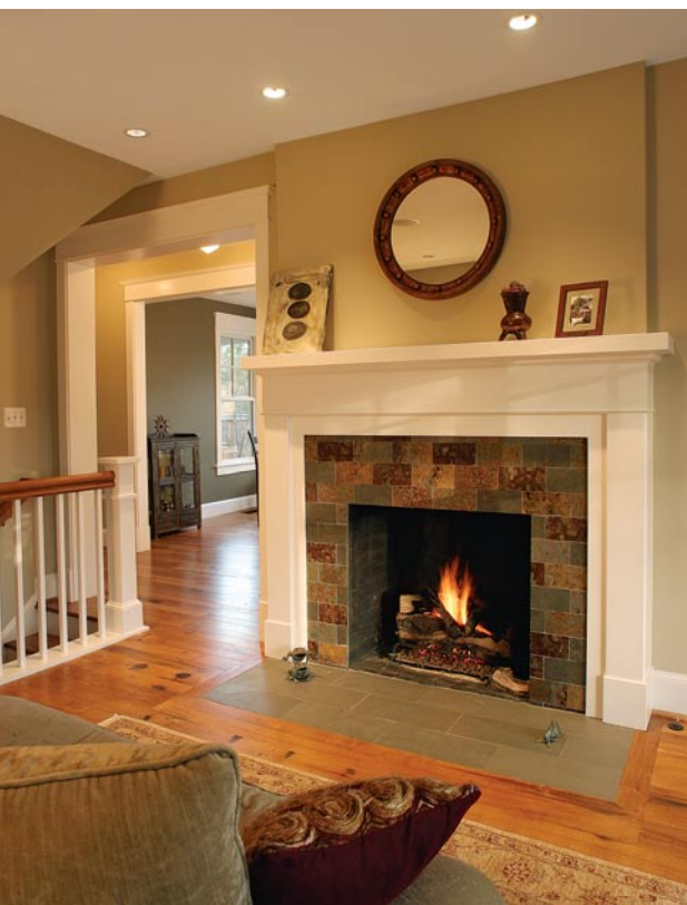
Keep it quaint, make it modern. Although it now burns gas instead of wood, with a new mantel and a tiled surround, the fireplace warms the house more than ever. Photo taken at C on floor plan.
