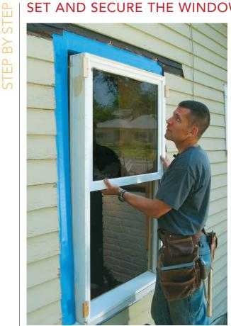
Set the window in the opening. Stop blocks help to align the window flush with the sheathing. Insert shims between the side of the window and the framing at the top and bottom to hold the window in place temporarily.
