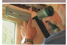
Apply the interior trim. Like the outside trim, the interior trim helps to secure the window in place. Use 18-ga. fasteners for the trim-to-window connection and 16-ga. fasteners for the trim-toframing connection. As shown in the photo below, you can use a reveal gauge to maintain a consistent reveal between the edge of the trim and the edge of the window jamb.
