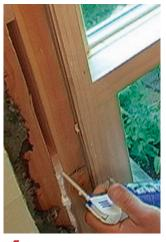
Fill the cracks. Use low-volume expanding foam to fill the void between the window jamb and the framing.
