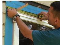
Center the window to the siding. Adjust the shims to center the window. Use a level to ensure that the window is plumb, then cross-measure and square the window to within 1/8 in. This should closely match the center of the rough opening. If the existing edge of the siding is out of plumb by more than ¼ in., you may have to taper the trim or cut the siding to make up the difference.
