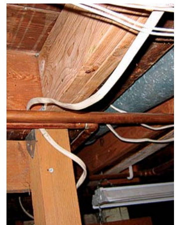
A work-in-progress shot shows utilities crowding the cantilever.
