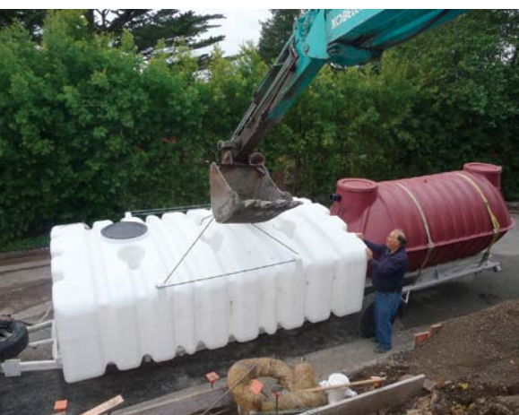
Ready for the rain barrel. Domestic water needs are partially supplied by rainwater stored in this 2500-gal. tank.
