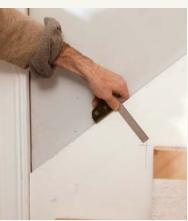
**Check the measurements.** Using a combination square, measure the distance from the top edge of the skirt to the upper riser mark. Next, compare the first measurement to the riser mark at the bottom of the stairs (photo right). Adjust the skirt position by trimming the level cut to compensate for any substantial difference (1/4 in. or more) between the two.
