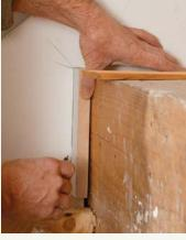
Locate the risers. With the notched inside skirt in place, level across the top landing to establish the height of the top riser. Scribe a piece of scrap riser to the skirt to establish the location of the face of the riser. Repeat at the bottom of the stairs. The two points, top and bottom, should be the same distance from the top of the skirt. They form the top and bottom points of the layout line.
