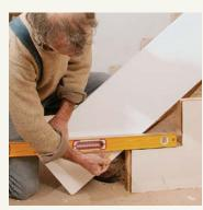
Repeat the process with the outer skirt. With the board in place, scribe the top vertical line against the drywall, then mark the level line at the bottom. The bottom plumb cut is made after the skirt is laid out.
