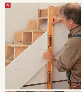
It's always good to check your work. Before cutting, tack the outer skirt in place, and make sure that the layout lines are plumb and level.
