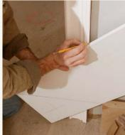
Scribe the bottom. Draw a level line across the skirt from the bottom stringer's first notch. Without changing the board's position, mark its intersection with the door casing, and draw a plumb line. Marking the waste side of the cuts helps you to visualize the finished skirt.
