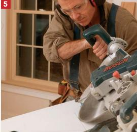
Miter first, from the front. With the skirtboard's top edge against the saw fence, cut the riser miters with a sliding compound-miter saw. (You also can use a circular saw.) Don't let the sawkerf extend more than ½ in. past the intersection of the tread line.
