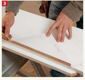
Keep it accurate with a template. Using the same pitch block made for the inner skirt, lay out the treads and risers. To avoid confusion, it's a good idea to mark the direction of the miters.
