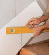
Mark the upper notch at the top of the stairs. First, draw a plumb line on the board. Next, measure up from the landing the height of one riser, and mark it on the plumb line. Draw a level line that intersects the plumb line.
