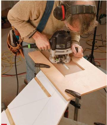
Rely on a simple jig. Make a jig from 1/4-in. and 1/2-in. plywood. The thinner plywood forms a base. The rectangular cutout in the 1/2-in. plywood top guides the base of the router. With a 3/4-in.-dia. straight bit, make an initial plunge cut in the jig base. At each riser position, the jig now can be lined up with the pencil lines and clamped into place. The depth of the dado should be half the thickness of the stringer stock.
