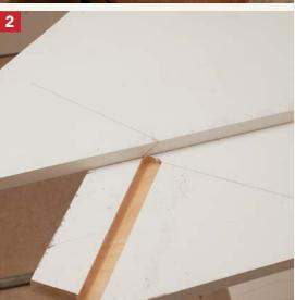
Start on the same page. Use the dadoed inner skirtboard as a layout template by aligning the outer skirtboard's top edge to the inner skirt's baseline and transferring each riser location to the outer skirt.
