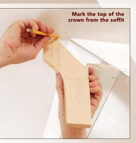
Tool of the trade. Take a 2-in.-long slice from the intended crown molding, and use it to trace the desired spring angle onto a 12-in. by 6-in. piece of MDF or plywood. Cut out the basic angle of the crown, then remove enough of the rest of the blank so that it's easy to hold with one hand. Place this spring gauge against the ceiling to mark the crown's position and to check the 1/4-in. reveal on the plywood soffit.
