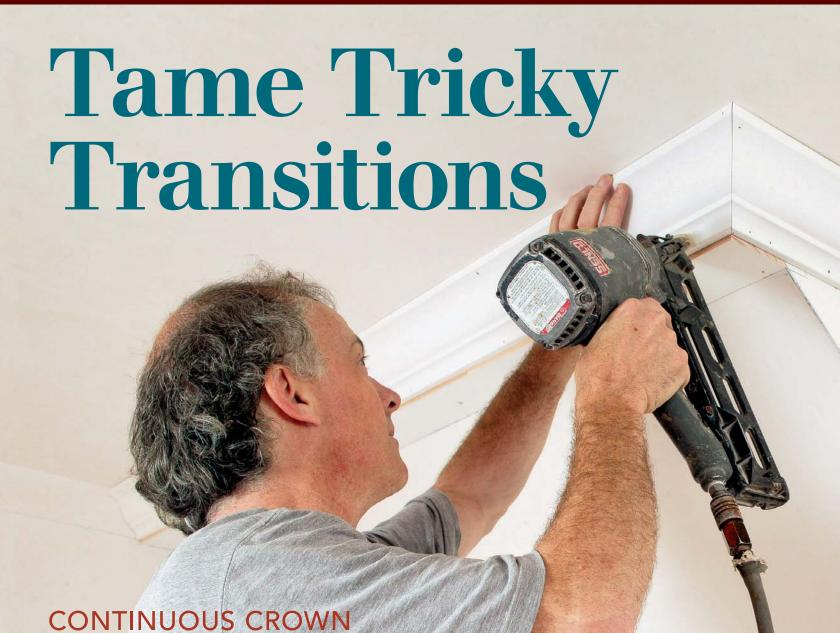
A line of crown molding can pass across a change in angle (such as at the top of the stairs) via a soffit. Built onto the angled wall, the soffit's width should be roughly equal to the widest part of the angle of the crown.
