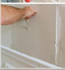
Prepare the grounds. With a flat bar, pop out the chair rail so that it's straight. Rip a few shims into 3/4-in.-wide strips. Measure the gap between the rail and the wall, then cut the fat end of the shims to match the gap. Insert the shims vertically, spaced at the width of the broad knife that you use. (The author's is 10 in. wide.) Tack them in place with a small nail.
