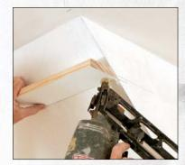
Snap lines, and install the soffit. Chalklines determine the lower position of the crown. The plywood soffit, beveled to the wall's angle, must be wide enough to create a surface perpendicular to the ceiling.
