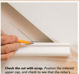
short point intersects the lower line. Repeat the process with the lower cap.
