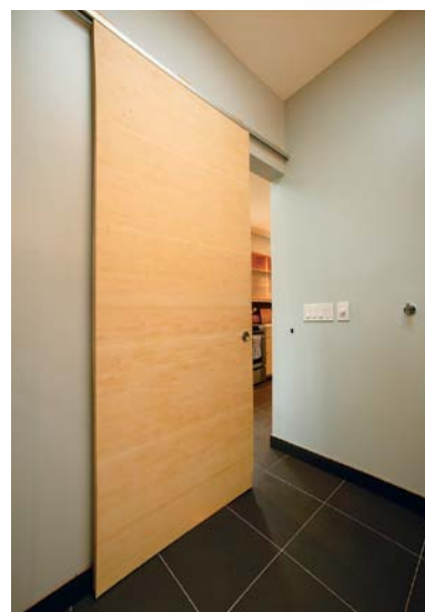
Space-saving door. Rather than take up valuable real estate with a swinging door, the author applied bamboo veneer to a 1½-in. slab of MDF and hung it from heavy-duty track hardware. The dense slab not only matches the cabinets, but it also keeps noise to a minimum.
