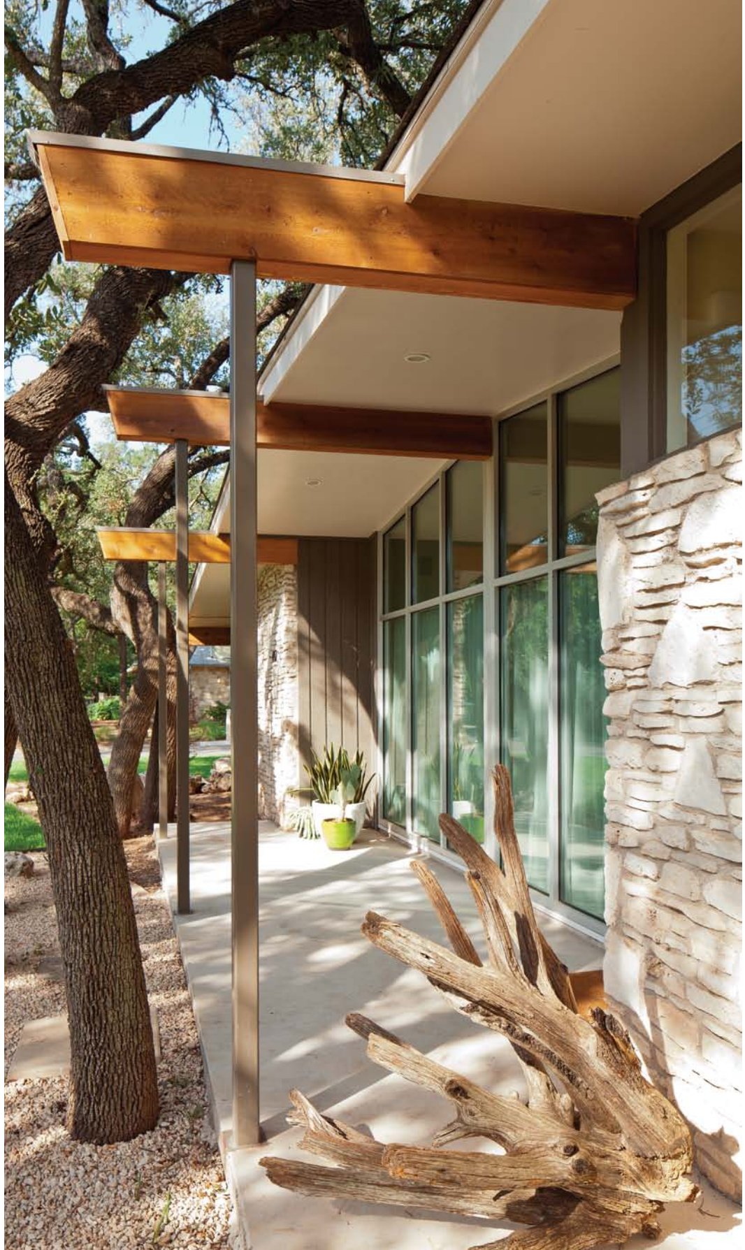
Use authentic materials. Most of Stenger's houses were built for clients using postwar FHA loans, which had certain aesthetic requirements regarding the use of masonry and other materials. Rather than apply imitative elements, as was the case with many homes of the time, Stenger built his houses with real masonry and local materials, and he made honest use of concrete and metal. Photo taken at E on floor plan.
