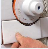
Curves require nippers. After installing as many full tiles as possible around the showerhead and mixing valve, you can use a pair of nippers to fit in the remaining tiles. Holding the tile in place, use a permanent marker to outline the area that needs to be cut. Carefully nibble up to the marked line with a set of tile nippers. The cuts don't have to be pretty; just get close enough so that the tile easily fits the open spot in the layout. The gap will be covered by the fixture's trim plate.
