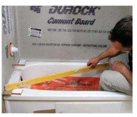
Know your tub installation. It would be nice if every tub installation were dead level, but that's rarely the case. Before you can begin the tile layout, lay a level across the top of each side of the tub. The bottom row of tiles can be cut to follow the contour of the tub or to account for high spots, so the goal here is to find the low point, which becomes the starting point for the rest of the layout.
