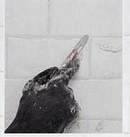
Pack and tool the joints. Once the grout has firmed up but before you wash down the tile, use the butt end of a Sharpie permanent marker as a grout stick to strike the grout joints. This packs in the grout tightly and makes the joint consistent.
