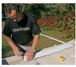
A stick tells the story. Cut a piece of wood for the vertical layout and another for the horizontal layout, each a bit shorter than the distance between tub and ceiling or wall and wall. Place the tiles one at a time, including a space for grout between each if the tile isn't self-spacing, and mark the layout on the stick.
