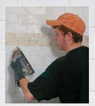
Spread and scrape. Use a margin trowel to load grout onto a rubber float, and then use the float to apply it to the wall. Spread the grout in broad, arcing strokes. Start with your arm extended, and pull the float toward your body. The first pass packs grout into the joints; the second pass scrapes away most of the excess.
