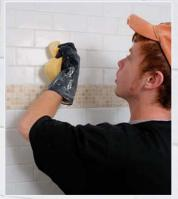
Wipe away the haze. Once the tile has been washed down and all excess grout removed, let everything dry for about 15 minutes, or until a light haze develops on the surface of the tile. Then use a clean cloth or quality paper towel to wipe the haze off the surface of the tile, buffing it to a finished shine.
