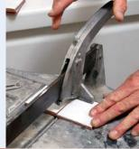
Score and snap. For all straight cuts, a basic snap cutter works quickly and makes a clean cut. Score across the top of the tile, then give the handle a quick bump with the palm of your hand to break the tile at the score line. If the cuts are difficult, small, or notched, a tile saw is a better choice.
