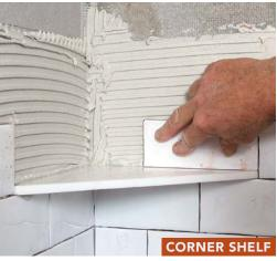
I typically make a corner shelf from a 12x12 stone tile. Here, I cut a piece of marble in half diagonally and then rounded over the edges with a rub brick. Installation is easy: Butter the back edge of the shelf with thinset and rest it atop a course of tiles. Trim the next course of wall tiles as needed. To keep water from pooling on the shelf, put a few temporary plastic wedge spacers under the shelf, all the way at the back of the corner, so that it sets up with a slight pitch.
